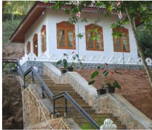
Newly constructed Seema Malakaya
